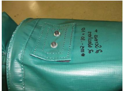
Secure the Velcro panel in place using the screws and washers provided/
