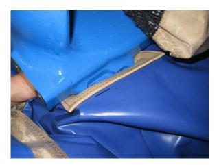
Photo-40: Slide gum rubber over synch marker
